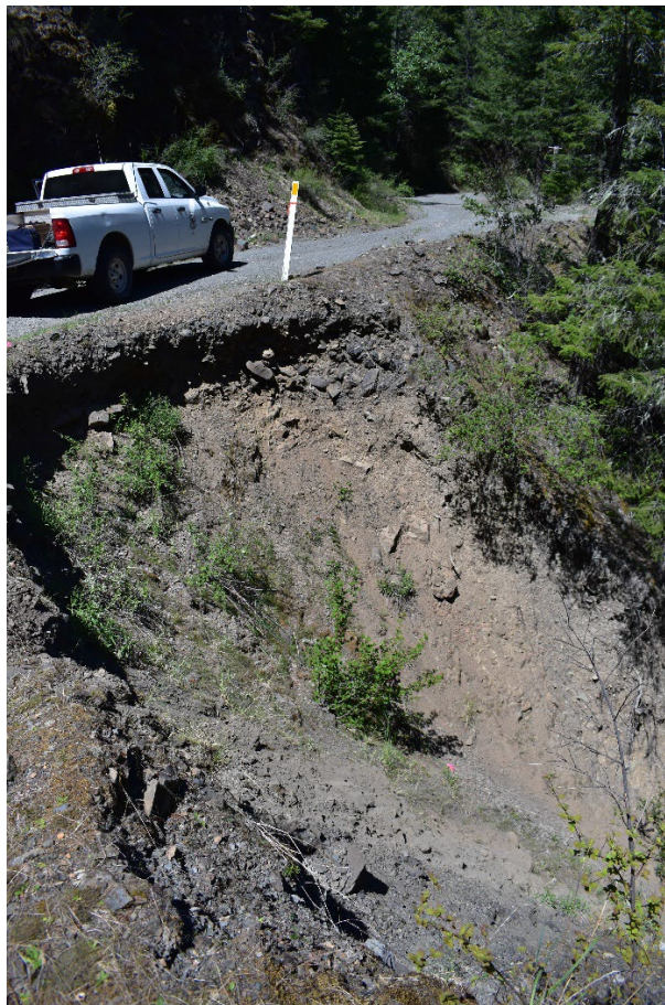
(Proposed Retaining Wall Site looking north)
